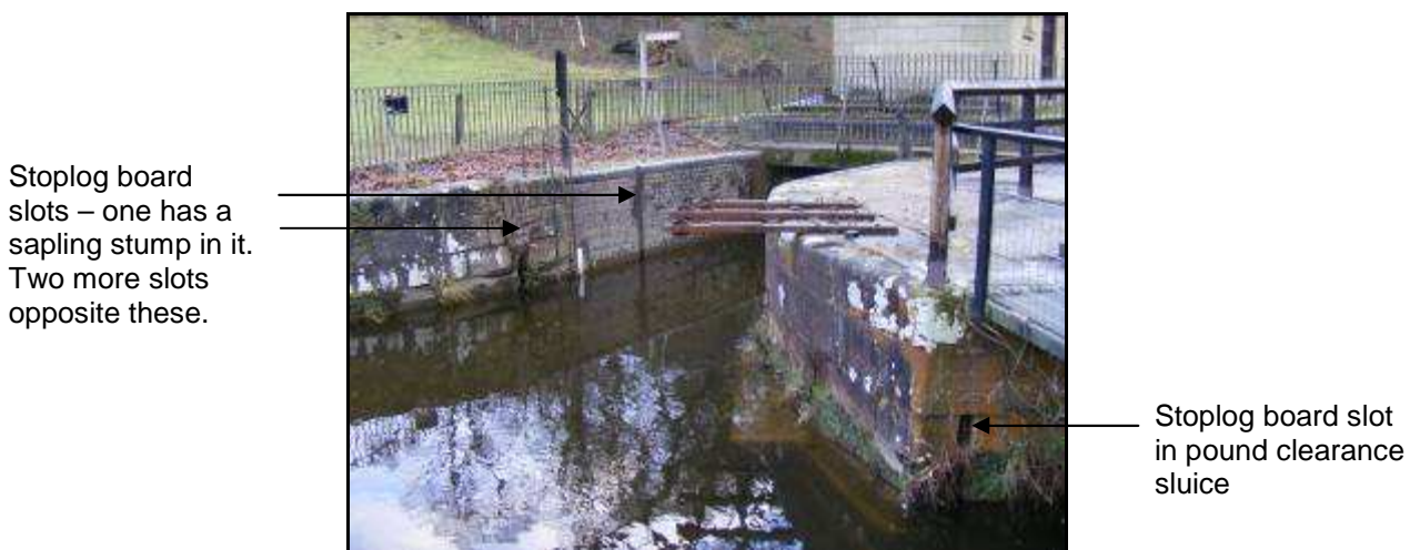
Figure 28 – Provision for stoplog boards in pound.
