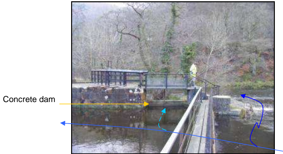
Figure 26 – Canal abstraction (left), pound clearance sluice (middle), River Dee (right).
