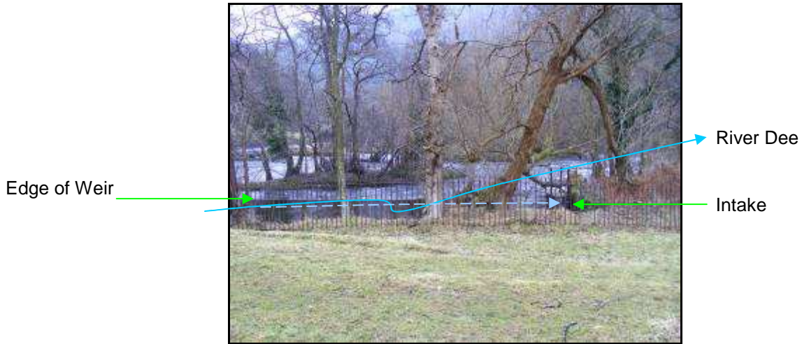
Figure 7 – Dee Valley Water screen and intake.
