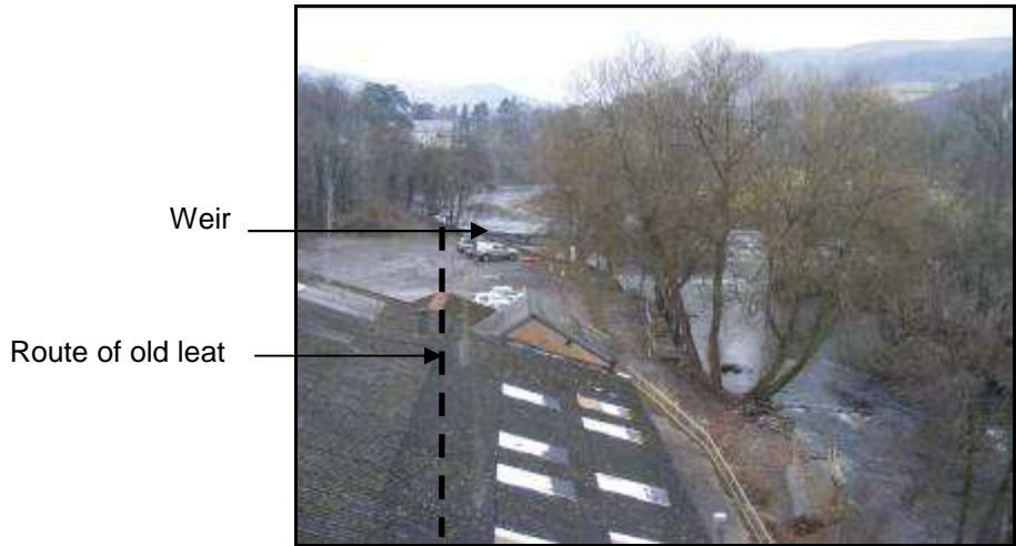
Figure 35 – View upstream from top floor of mill.
