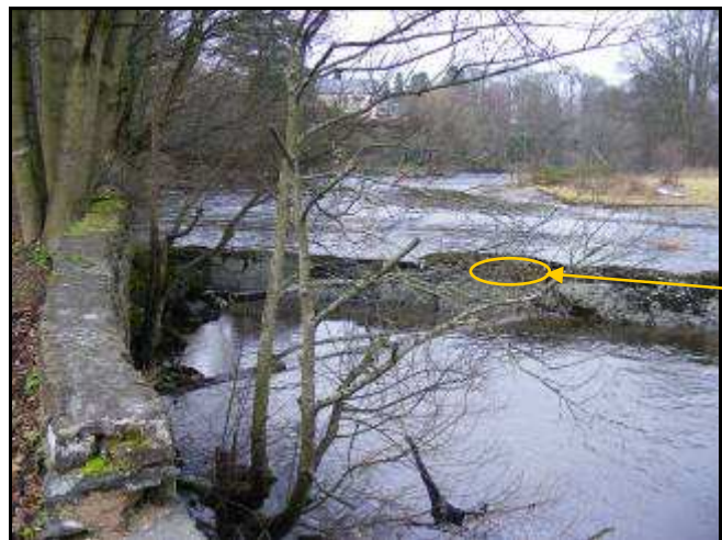
Figure 36 – Intact part of weir where it meets the western bank.
