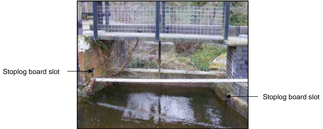
Figure 29 – Close up of stoplog board slots in pound clearance sluice.
