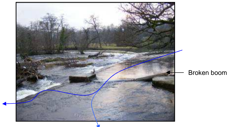
Figure 22 – Boom (broken) just upstream of British Waterways intake.
