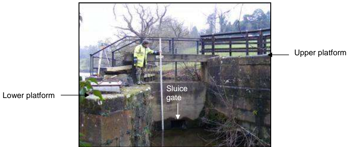
Figure 27 – Pound clearance sluice with sluice gate in concrete dam.
