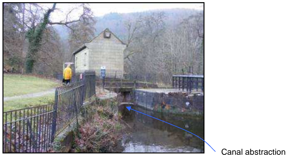
Figure 25 – pump house, pond and footpath.
