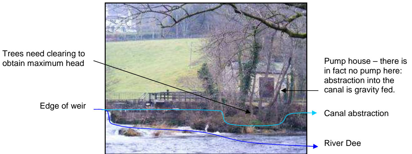
Figure 24 – Existing British Waterways installation, taken from other side of river.
