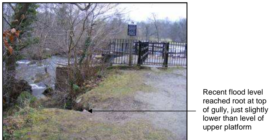
Figure 31 – Recent (last 20 years) flood level according to British Waterways operative.
