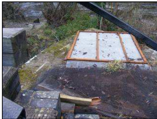
Figure 30 – 10 mm and 4 mm screens used for part of the year.
