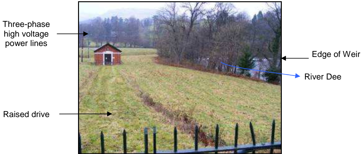
Figure 10 – Dee Valley Water building.
